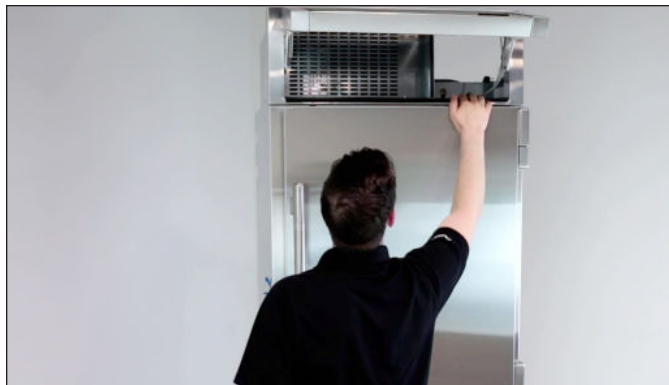
FIG. 3. Be sure to inspect the rainshield.
