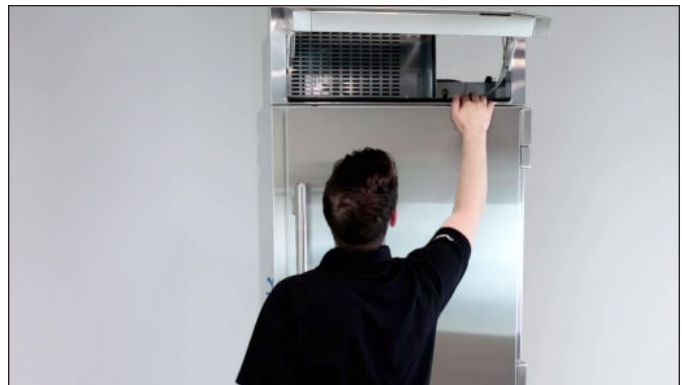
FIG. 3. Be sure to inspect behind the rainshield.
