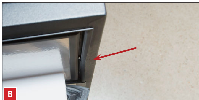
FIG. 3B. Bowed gasket channel.
