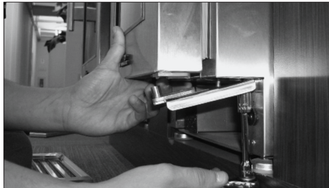
FIG. 5. Install the 90° door hinge. Do not fully tighten hardware.
