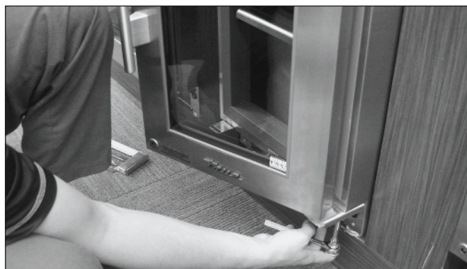
FIG. 6. Tighten the bottom hinge hardware after adjusting the door alignment.
